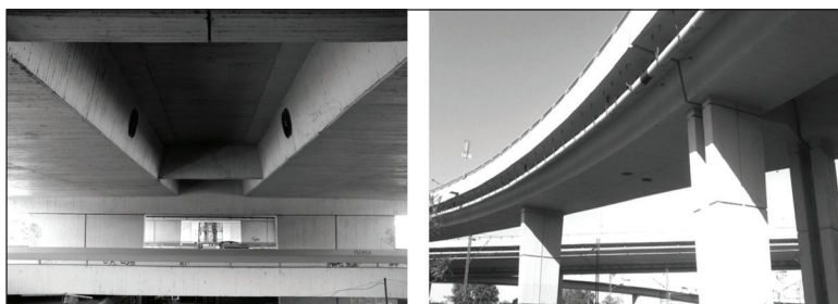
Figure 2. Photographs of the Mostar Interchange
