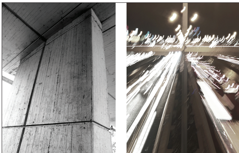
Figure 3. Photographs of the Mostar Interchange
