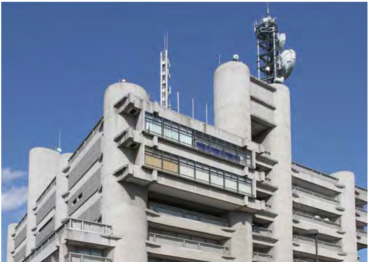
Figure 1. Kenzo Tange & URTEC, Yamanashi Press and Broadcasting Centre, Kofu City, Japan, 1964-1966; Tange Associates, renovation, 2015-2016. Exterior view from south. © Ana Tostões, 2017.
