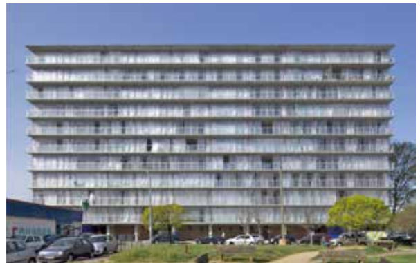
Figure 1. Block G exterior before and after the transformation photo credit © Philippe Ruault
