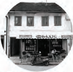
residential and commercial building
