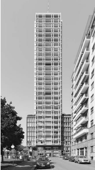
Figure 6: Luigi Mattioni, E. and E. Soncini; Torre Breda, Milan, 1950-55; photographer Maurizio Montagna.
