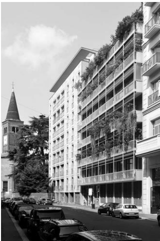
Figure 9: Guglielmo Mozzoni, Luigi Ghidini; Building in Via Fatebenefratelli, Milan, 1952-53; photographer Daniele Zerbi.
