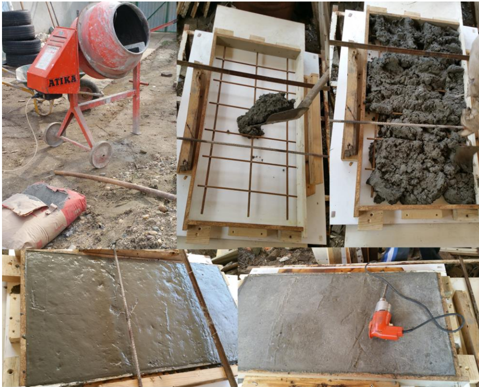
Fig. 8 Embedding concrete
