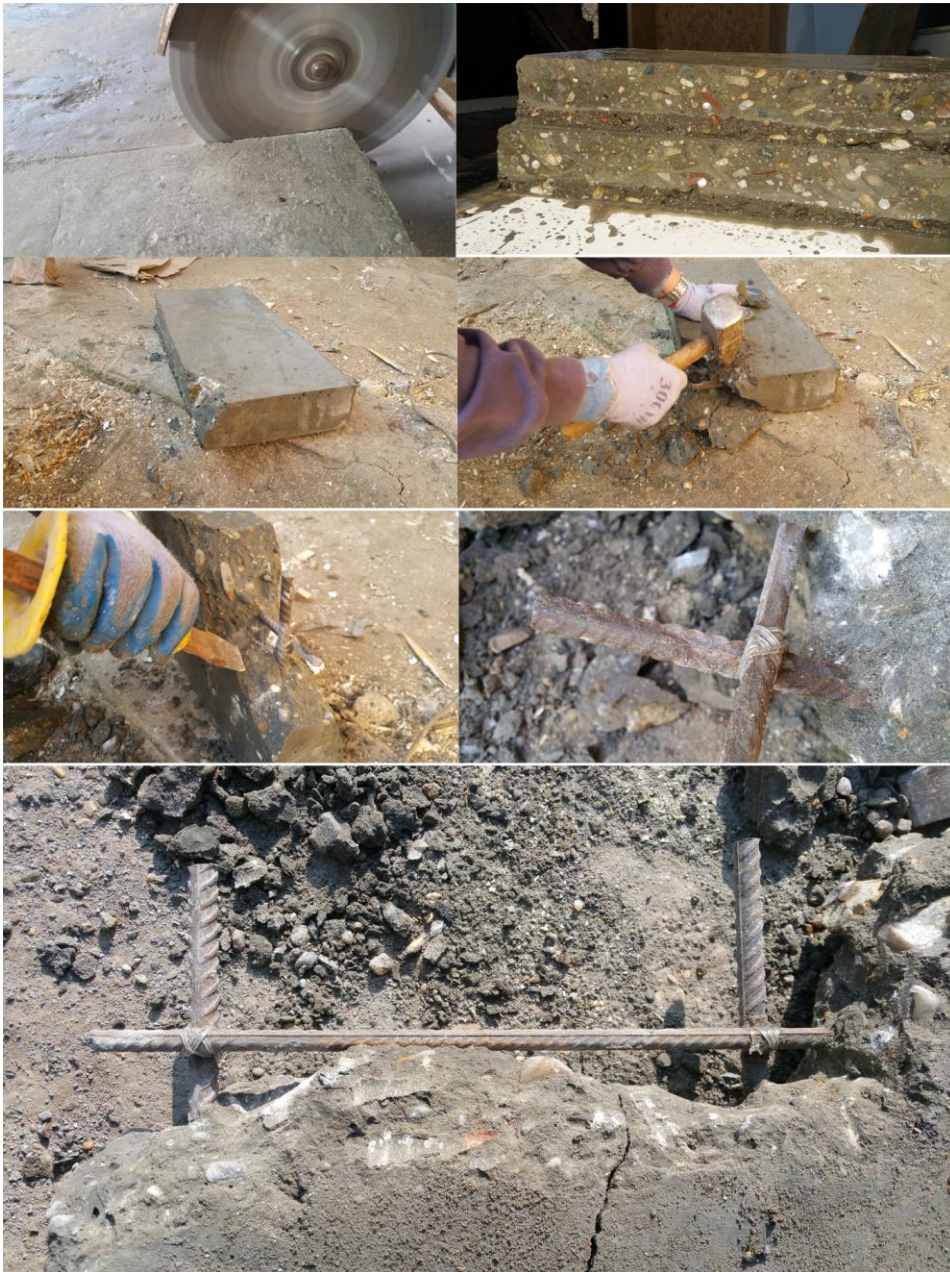
Fig. 9 The demolition and visual detection
