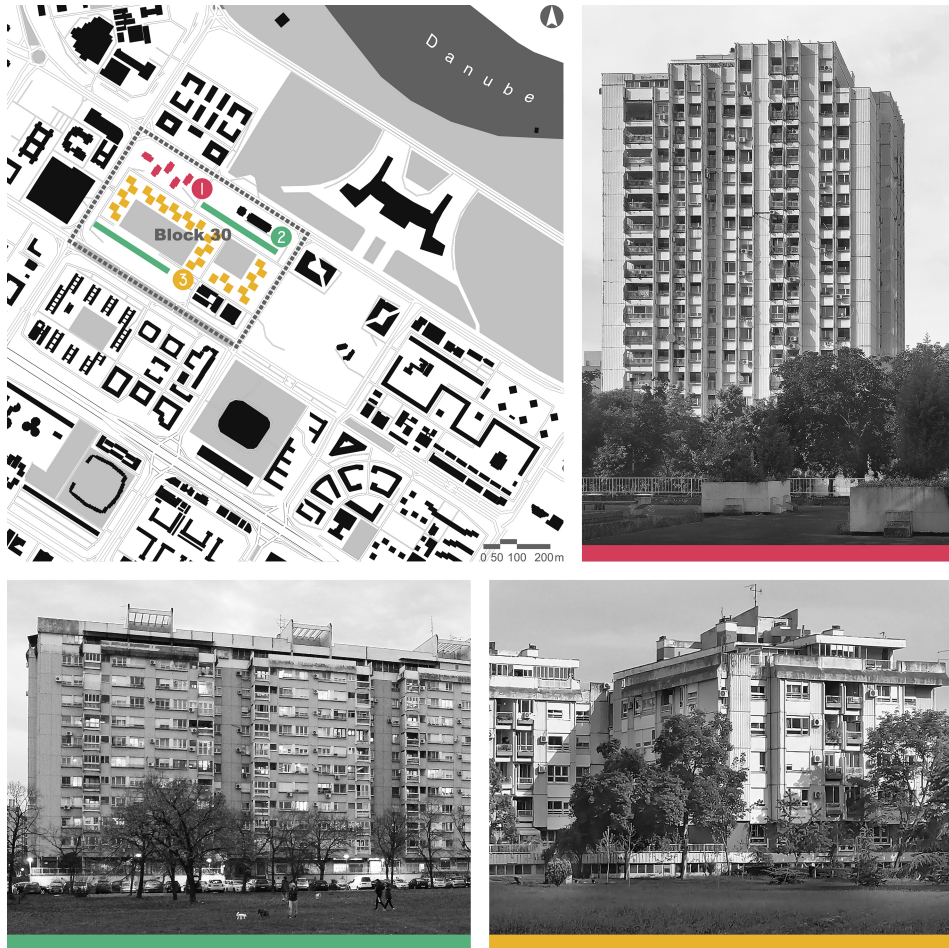
Figure 1: Block 30 – Borders & Building Types Marked in the Urban Tissue of New Belgrade and Representatives of the First, Second, and Third Type of Residential Buildings (left-to-right, top-to-bottom). Source: Author, 2023
