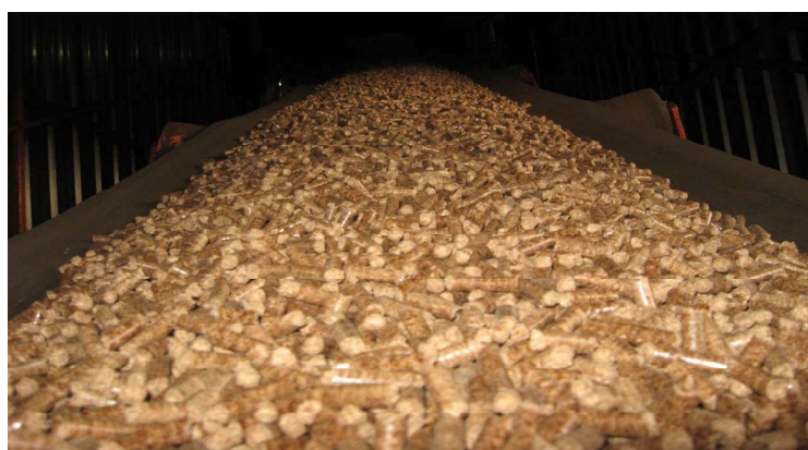
Figure 2 - Pellets (biomass) as a fuel in a local boiler station "Simiceva" of PUC " Beogradske elektrane" in Belgrade.
