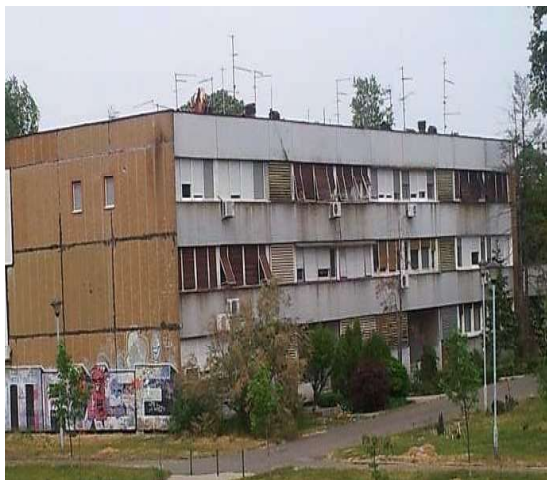
Figure 5 - The building in the street Nehruova 178, Block 45 in New Belgrade.
