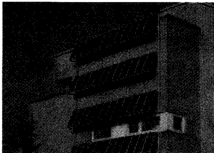
Fig. 1b. Facade "standoff" PV system
