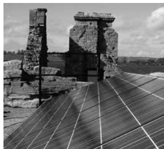
Figure 2. Photovoltaic panels in Crichton Castle Scotland
