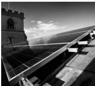
Figure 1. Photovoltaic panels on the roof of the nave at Wing All Saints, Buckinghamshire
