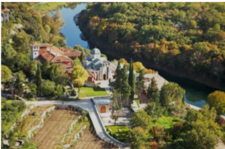
Figure 21: Monastery Tvrdoš, existing state.
