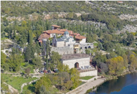
Figure 19: Monastery Tvrdoš, existing state.
