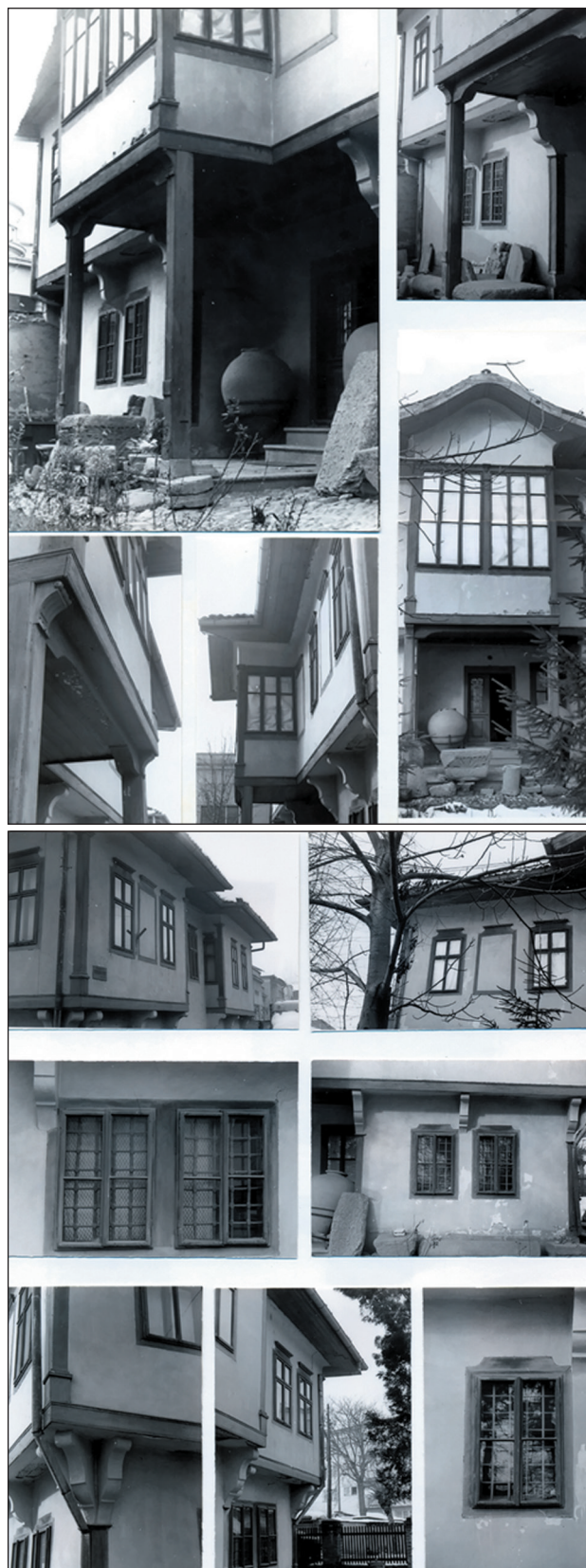
Picture 3. Photos showing the existing condition of characteristic architectural elements (entrance overhang of „divanhana“, double bay windows- „erker“, entrance part, roof eaves and facade walls) before reconstruction
