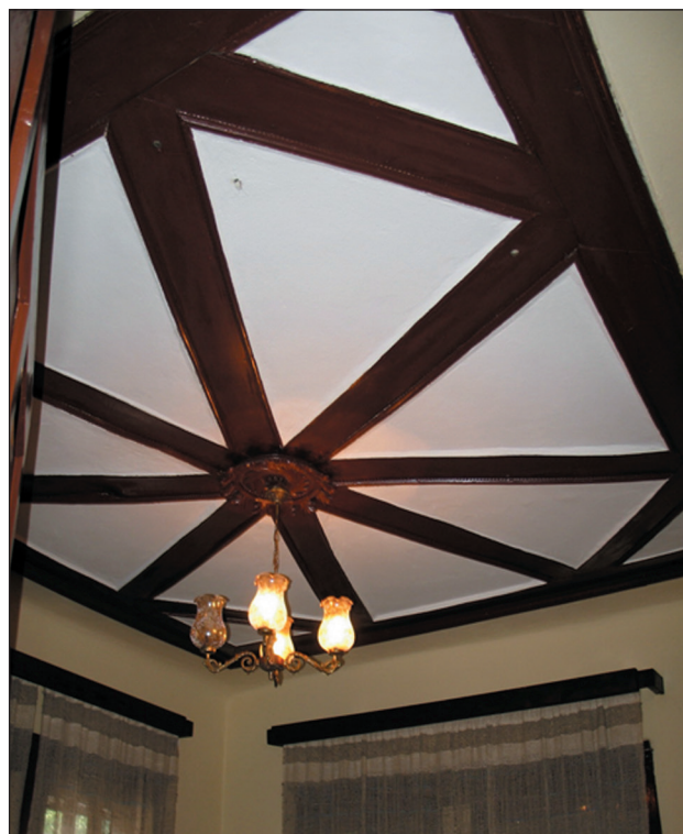
Picture 7. A segment of the ceiling construction
