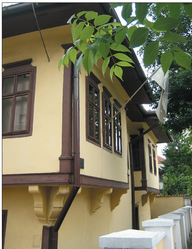
Picture 14. A segment from the street-side facade with typical double bay windows-„erker“
