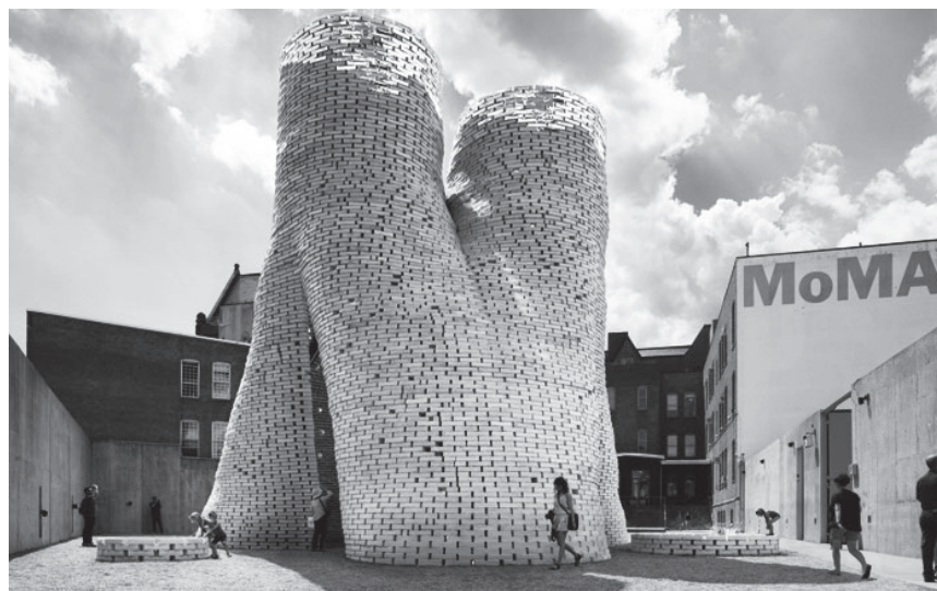
Fig. 10. “The Living” (New York-based designed practice group), 12m-high Circular Tower made of biodegradable bricks for MoMA PS1’s annual Young Architects Program, 2014.
