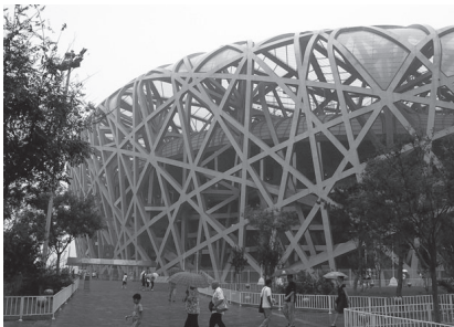
Figure 4. Herzog and De Meuron, Olympic Stadium, Beijing, 2008. General view.
