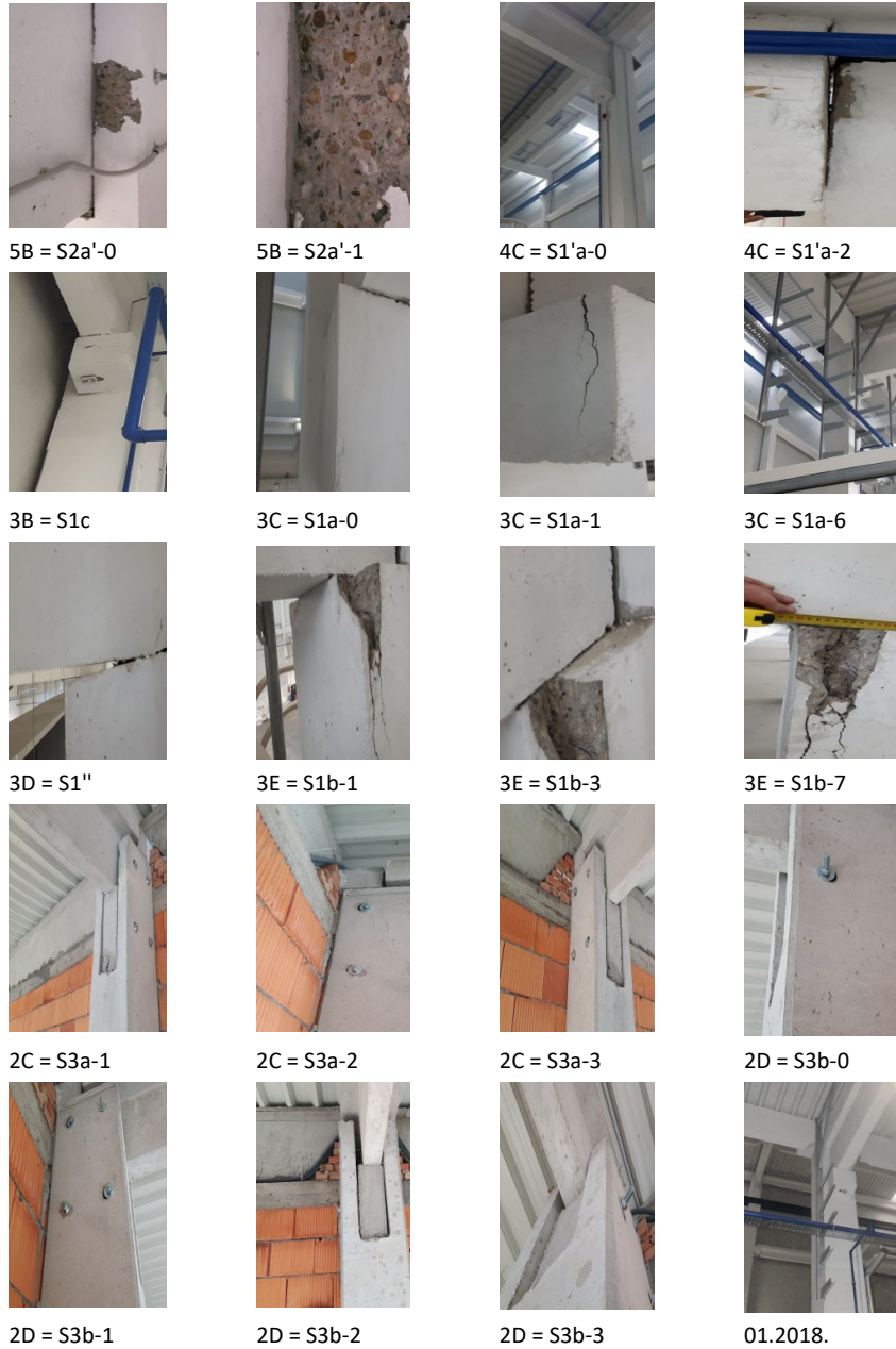
Figure 2 – VPF hall nonconformities selection
