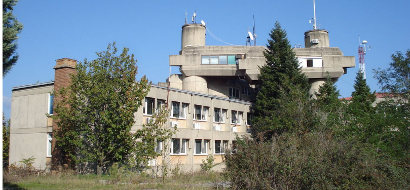
Figure 1. Macedonian Hydrometeorological Service building
