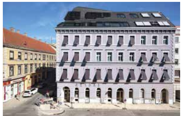
Figure 3. Roll-out sunscreen attached to the windows to reduce the cooling demands.
