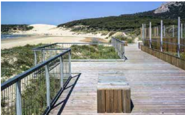
Figure 3. Structure of the walkway over the dune of the coastal edge. Leisure areas and geometry translation of the shape of the cardo Source: IAPH
