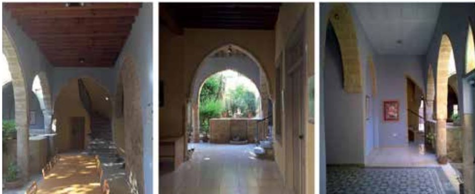
Figure 2. Building complex under study. (a) East facade showing sahnisi on the first floor, (b) semi-open spaces (iliaki) and courtyard and (c) north facade.
