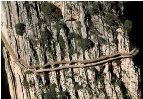
Figure 1. Aerial view of the two footbridges
