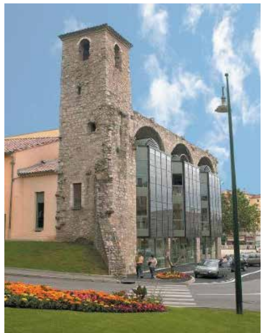
Figure 1. View of the building where the integration of the PV-system in the three bays can be seen.
