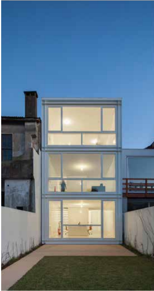
Figure 3. House— rear façade Copyright: Photographs by José Campos
