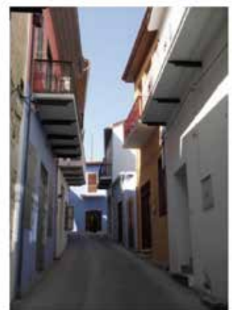
Situation after works
