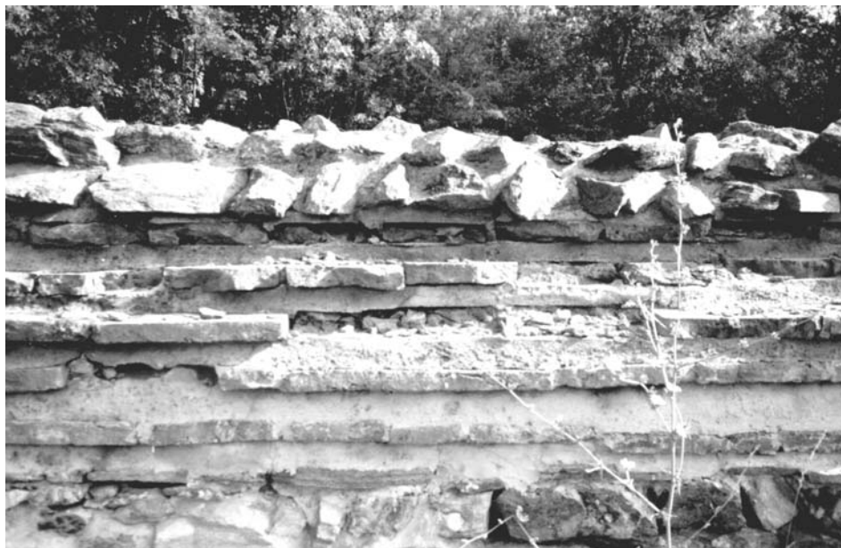
Fig. 2. Typical example of degradation - part of wall of a so-called double basilica from the archaeological site of Caričin Grad, extended with contemporary materials
