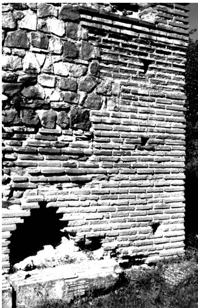
Fig. 3. Detail from the fortification of Gamzigrad (Felix Romuliana) where bricks produced in a different way were applied in different phases of conservation work
