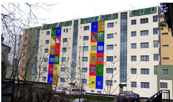
Fig.6. Court yard facade after refurbishment, residential building, Cvijićeva str. 112-120
