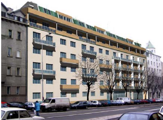
Fig.4. Street facade after refurbishment, residential building, Cvijićeva str. 112-120
