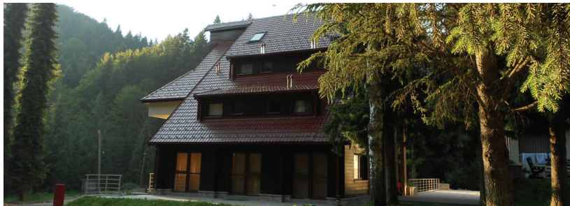
Figure 4: One of the new, expanded buildings in the Goc teaching base (Serbia). Designed in 2013, constructed in 2015. Authors: A. Videnovic, D. Radonjic, D. Danilovic, architects. (Photo: A. Videnovic)
