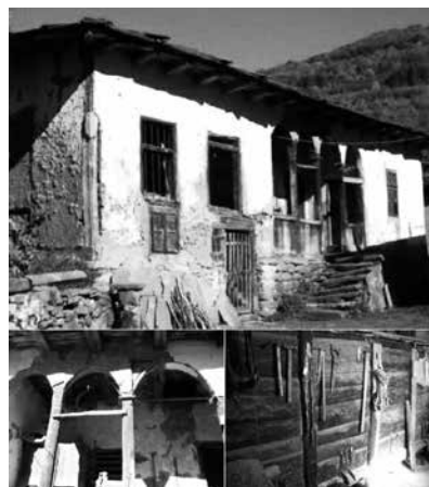
Figure 3. The house of Desimir Kostić, 1900, Village of Brlog (the entrance façade and details of the porch with arches and wooden storage elements called preseci , below, credits: G. Ljubenov)
