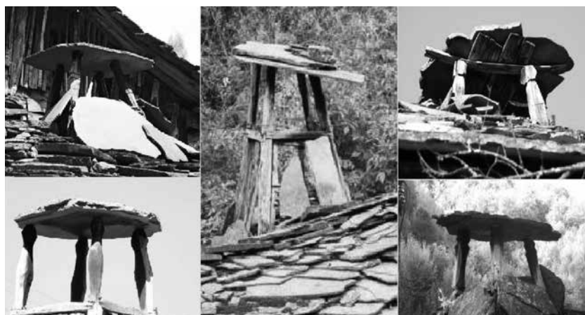
Figure 4. The chimneys caps (called kvačke ), Villages Dojkinci, Brlog, Gostuša and Topli Do
