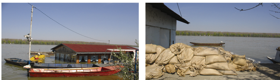
Fig. 3. Emergency repairs with sandbags and flooded restaurant on the Zemun waterfront in Belgrade at high water levels in 2006 (Lazarevic Bajec, 2009)
