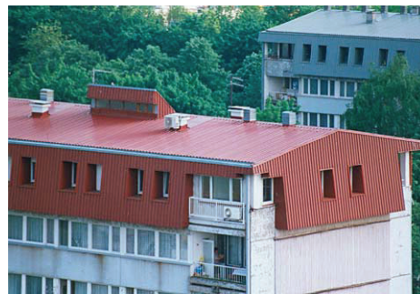
Figure 4: Typical building after attic annex
