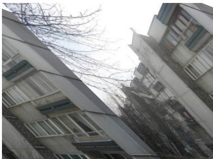
Figure 3: Typical building before attic annex
