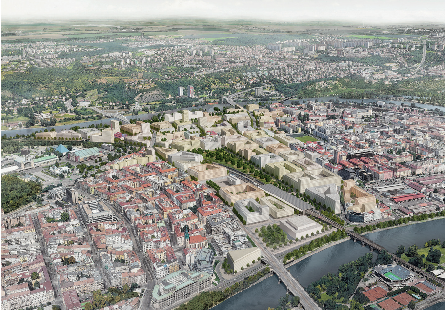
Fig. 12: Visualization of the future development of the Bubny railroad area /Source: Institute of Planning and Development, IPR Praha
