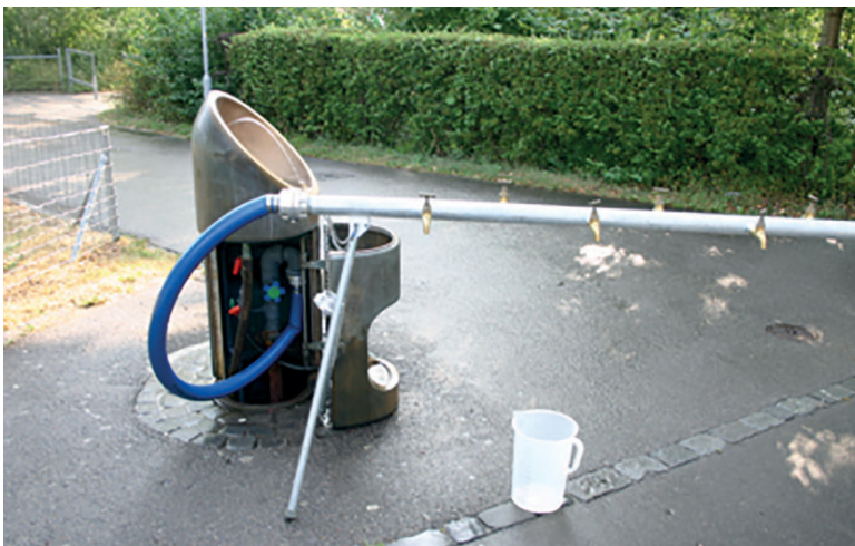
Figure 4: Emergency water fountain in the city of Zurich. Above: in normal mode; below: in emergency mode. © Wasserversorgung Zurich
