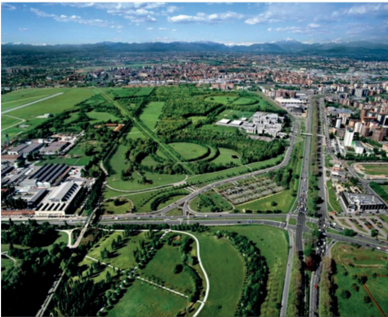
Figure 5: The current state of the core park area.
