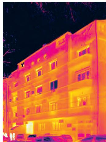
A residential building with massive façade brick walls without thermal insulation. The thermal image shows heat losses through façade walls particularly intense at horizontal reinforced concrete ring beams and parapets, resulting from reduced wall thickness. There is remarkable heat loss at the display window on the ground floor and particular original wooden windows.
