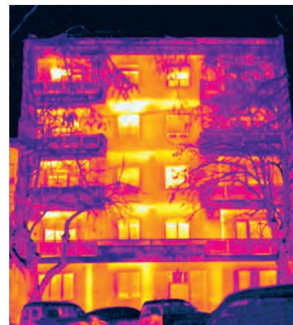
A residential building with massive façade brick walls without thermal insulation. The thermal image reveals noticeable heat loss through façade walls, particularly at horizontal and vertical reinforced concrete ring beams and cantilevered terraces. The original façade fenestration reveals intense heat losses at frame connections and roller shutter boxes.
