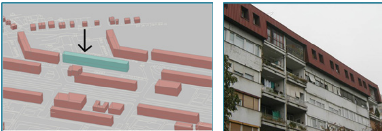
Figure 1: Location (left) and appearance (right) of the building in Konjarnik settlement
