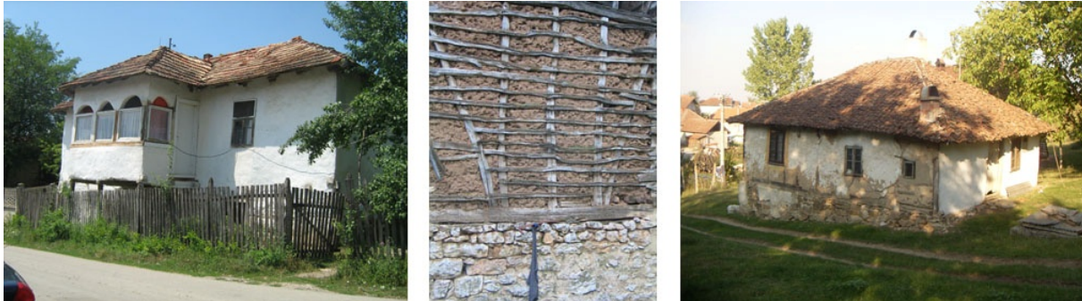
Fig. 3 Example of bondruk style houses from South East Serbia (left) and East Serbia (right) and detail of the building technique (center)
