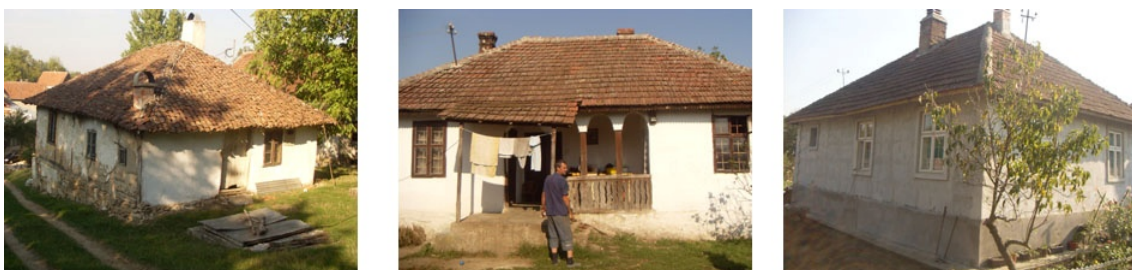
Fig. 7 Different treatment and usage of traditional bondruk style houses in Serbia: abandoned (left); in use with minimal interventions (central), improved with contemporary thermo-insulating materials (right)
