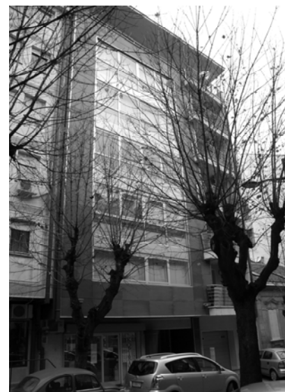
Figure 14. The combination of composite materials as a facade cladding and a large glass surface, Building in Dušana Bogdanovića Street, Belgrade, MetricCo-architectural team, Street appearance of the building (Ivanović-Šekularac, 2010)
