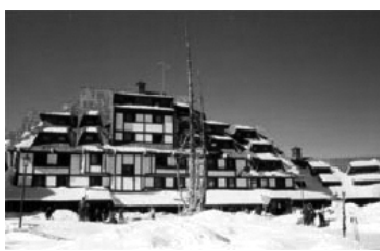
Figure 3. Wood in combination with a full wall carcass as a facade cladding and roofing, Grand Hotel, Kopaonik ( http://www.kopaonik.net/main.php?case=smestaj&leng=ser )
