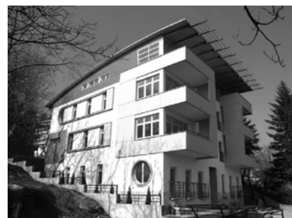
Figure 6. The facade is created as the combination of wood, composite materials and painted wall surfaces. Multi-family residential building "Condominium 41-7", Velisava Vulovića Street, Dedinje, Belgrade, architect Mustafa Musić, 2008., The appearance of the building ( http://www.enterijermagazin.com/index.php/mustafa )
