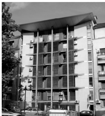
Figure 9. Wood as an element of the facade cladding in combination with a facade of artificial stone, Residential building, Kumanovska Street, Belgrade, 2000. Branislav Mitrović, The appearance of the building (Ivanović-Šekularac, 2010)
