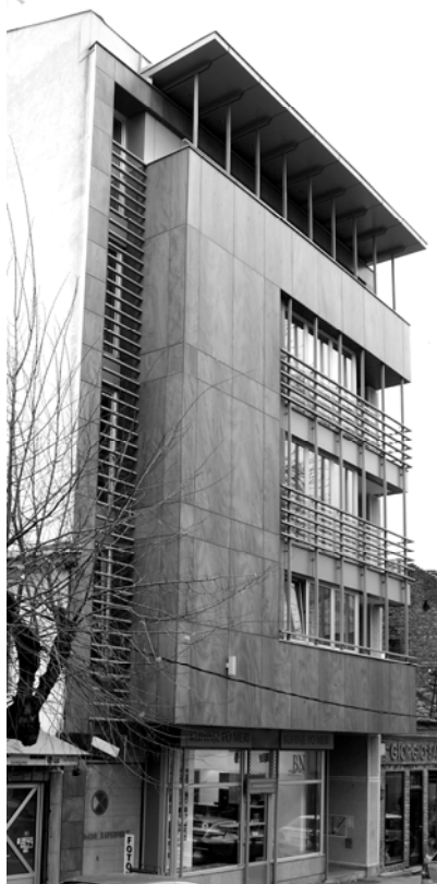
Figure 11. Composite material as a facade cladding in combination with glass and metal on the facade, Building in Jagićeva Street, Belgrade, Street appearance of the building (Ivanović-Šekularac, 2010)
