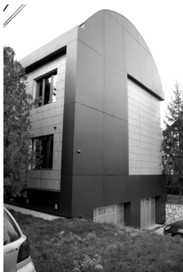
Figure 15. An example of reconstruction of the facade by placing the composite material as facade cladding, Building in Aleksandra Stambolijskog Street, Belgrade, Street appearance of the building (Ivanović-Šekularac, 2010)
