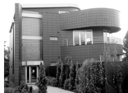
Figure 13. Composite material as a facade cladding, House on two corners, Mihajla Avramovića Street, Dedinje, Belgrade, architects Maša Bratuša and Lav Bratuša, 2006. The street appearance of the building (Ivanović-Šekularac, 2010)
