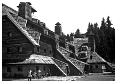
Figure 5. Wood applied as a wall, facade and roof covering; organic approach to architecture, Mountain House "Rtanj", architect M. Đorđević, Kopaonik, ( http://www.rtanj.com/wp-content/uploads/2008/10/image025.jpg )
