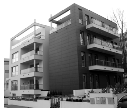
Figure 12. Composite material as a wooden facade cladding in combination with painted facade walls, Apartment building, Velisava Vulovića Street, Dedinje, Belgrade, 2008. The appearance of the building (Ivanović-Šekularac, 2010)
