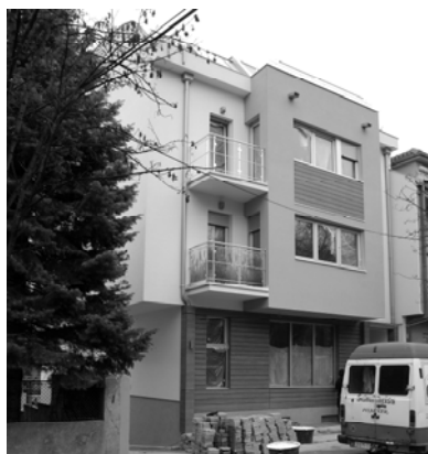
Figure 10. The combination of composite materials and painted wall surfaces on the facade, Residential building in Gospodara Vučića Street, Street appearance of the building (Ivanović-Šekularac, 2010)
