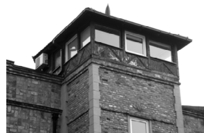
Figure 7. The combination of wood and brick as a facade lining, Milovana Marinkovića Street, Voždovac, detail of the building – the tower covered with wood (Ivanović-Šekularac, 2010)
