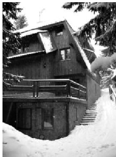
Figure 4. The combination of stone and wood as a facade cladding, "Paraglajder" Apartments, Kopaonik ( http://www.kopaonik.net/main.php?case=smestaj&leng=ser )
