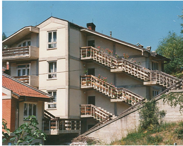
Figure 6. Multi-family residential building where each apartment has a separate entrance. Foreign experiences in the late 1970s in Crna Trava.
