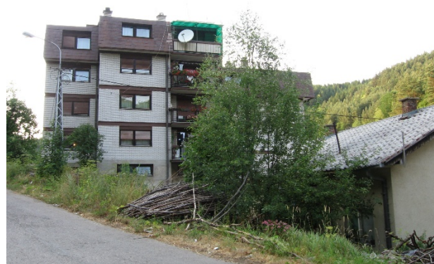
Figure 5. The facility for the needs of health and child care workers, built in the 1980s. Urban architecture in a rural landscape. (Crna Trava)
